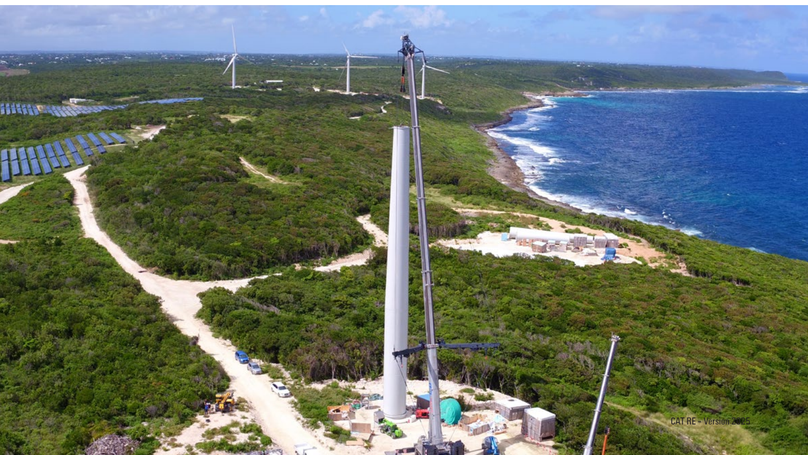
Installation work with the main crane on a LEITWIND wind turbine of the type LTW80 1.65MW Typhoon
