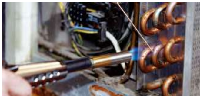
Brazing in air-conditioning and refrigeration technology
