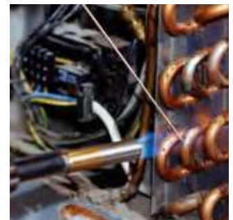
Brazing in air-conditioning and refrigeration technology
