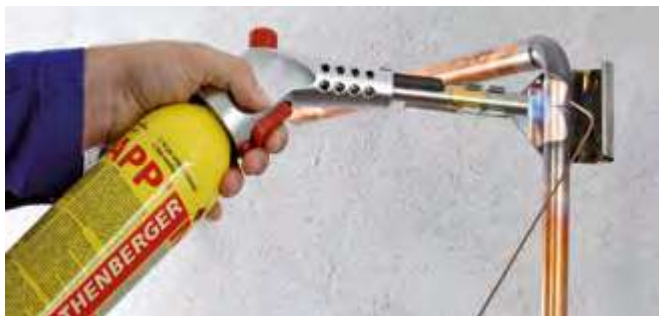
Brazing in gas installation
