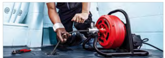
Cleaning of floor drain with 13 mm spiral
