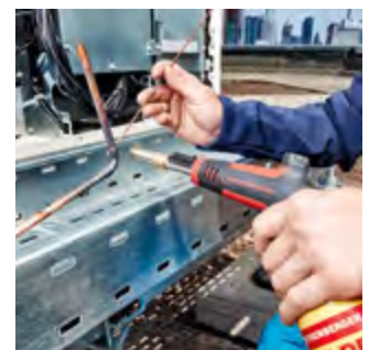
Brazing in air-conditioning and refrigeration technology
