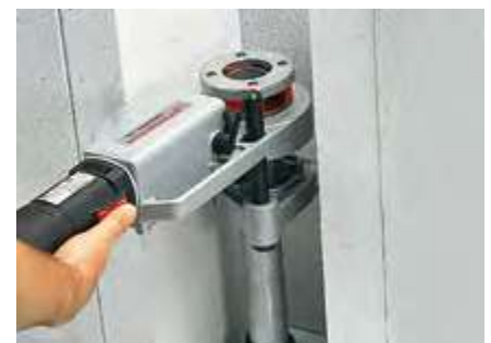
Work in confined spaces
