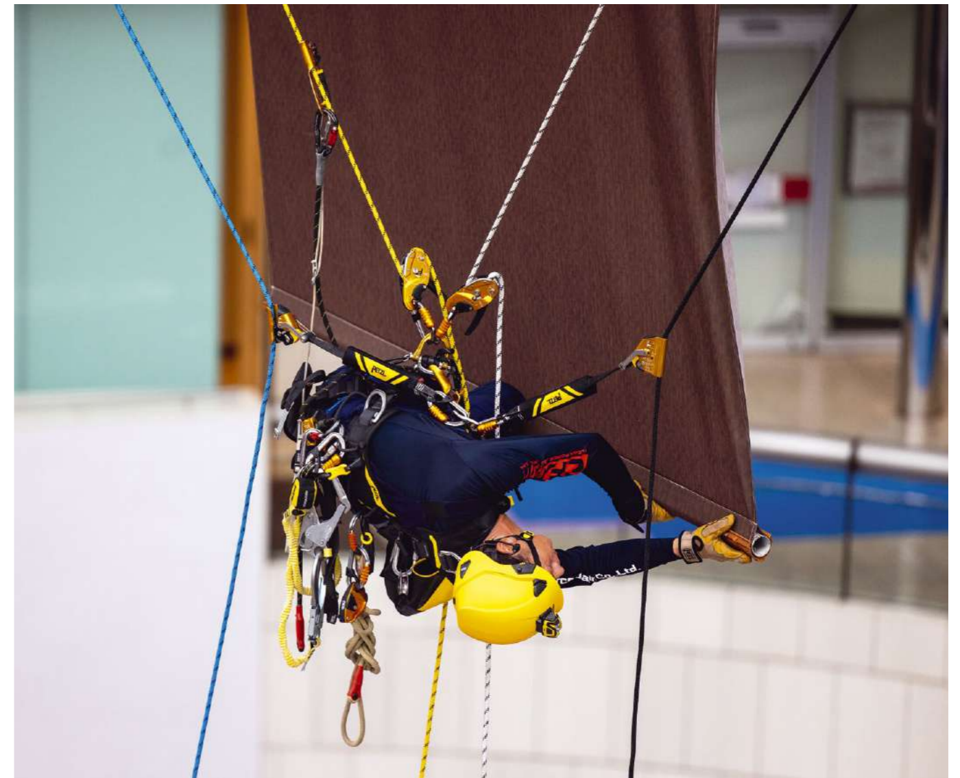
Rope access work at the Tokyo Metropolitan Theater. © 2025 Petzl Distribution - Lafouche - Tokyo Metropolitan Theater - Clean Force Japan
