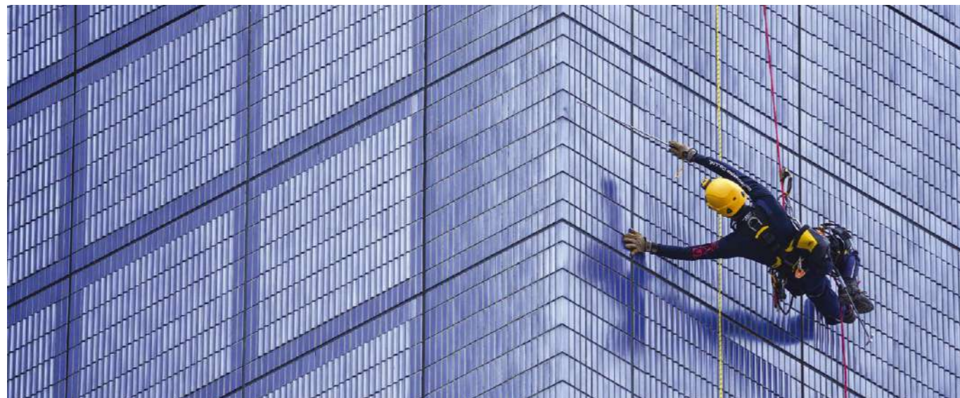
Rope access work at the Tokyo Metropolitan Theater
