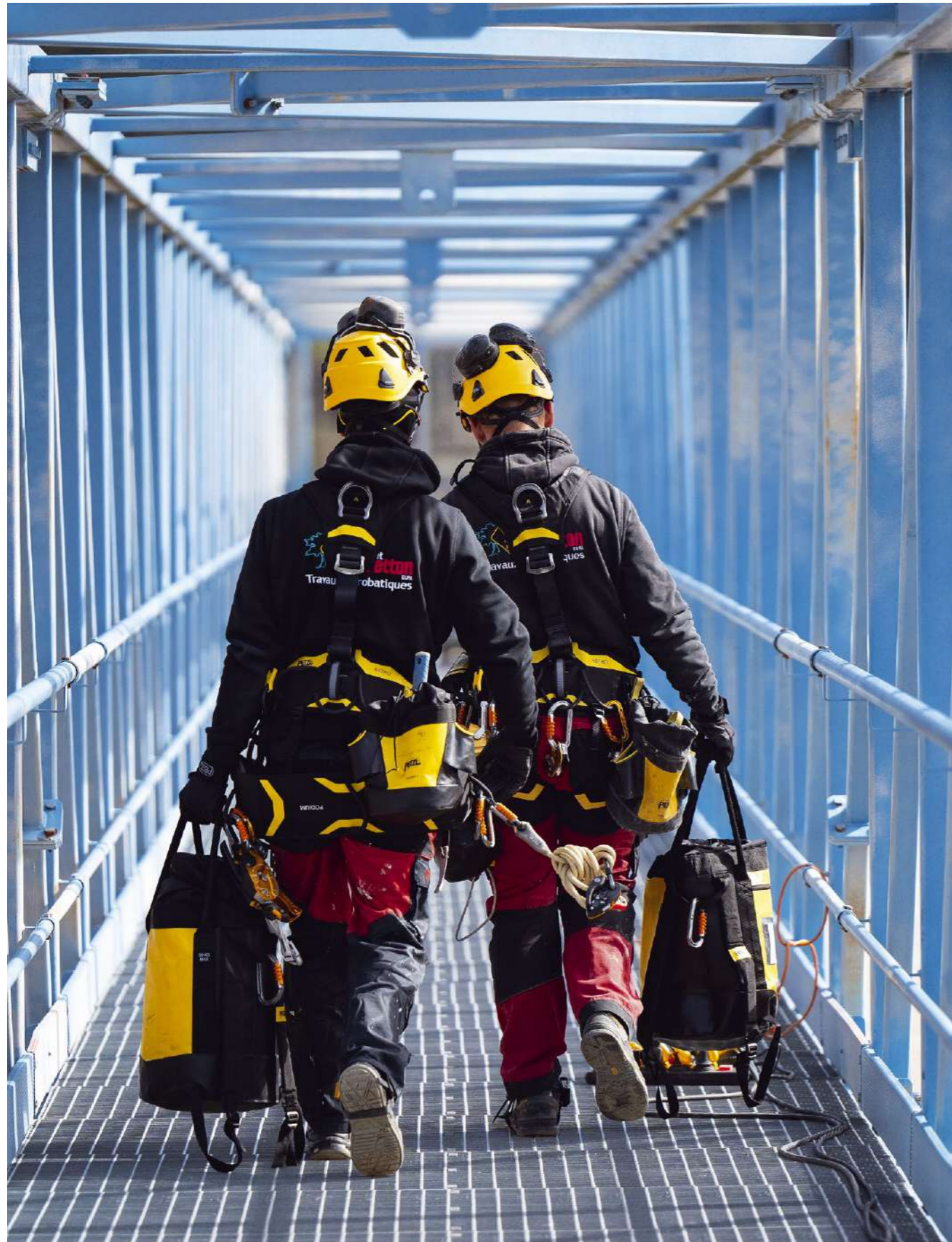
Rope access work on Barrage du Rouchain, France.
