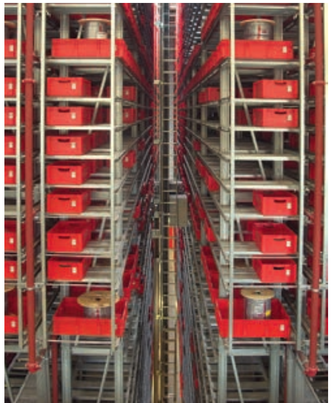
Small parts warehouse
